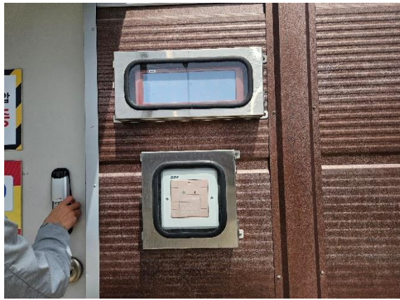
[Emergency manual activation panel]
