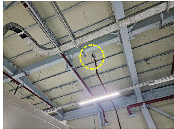
[Discharge nozzle in the substation]
