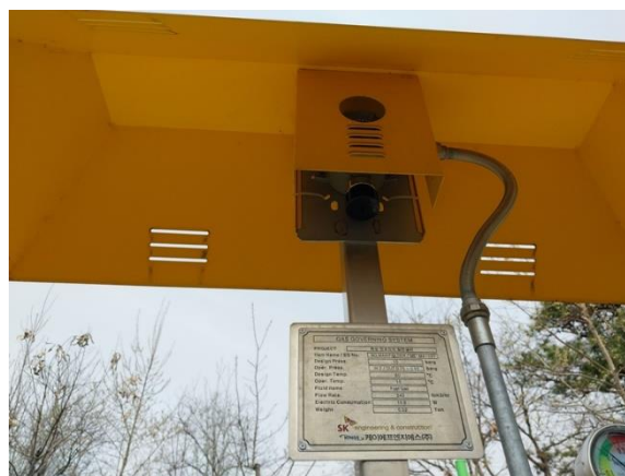
[Gas leak detector]
