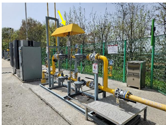
[Gas leak detector]
