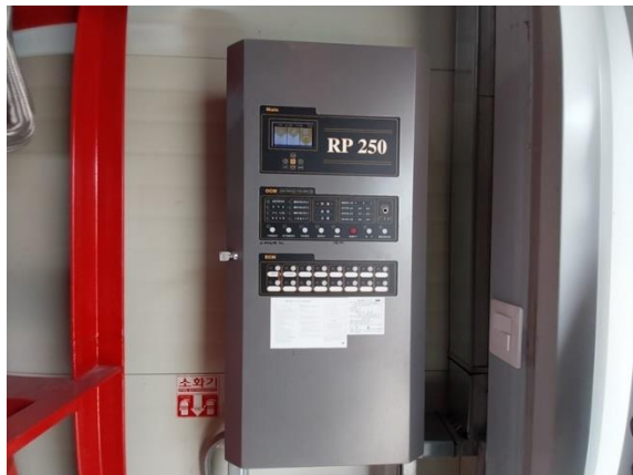
[Fire alarm control panel in the agent room]
