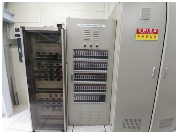
[Gas leak alarm system]
