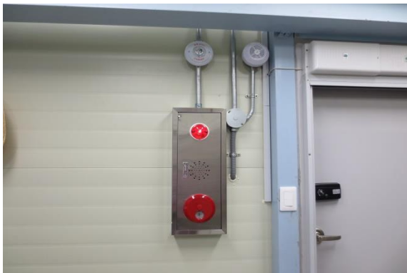
[Manual fire alarm push button]
