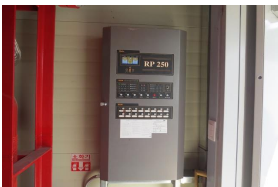
[Fire alarm control panel in the agent room]
