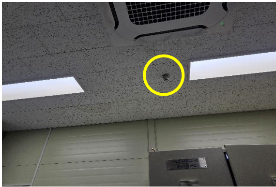
[Discharge nozzle in the control room]
