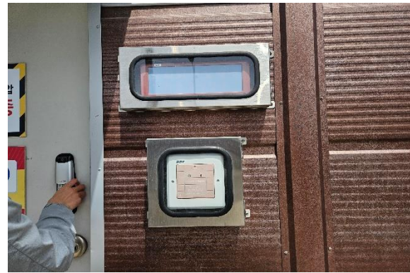
[Emergency manual activation panel]
