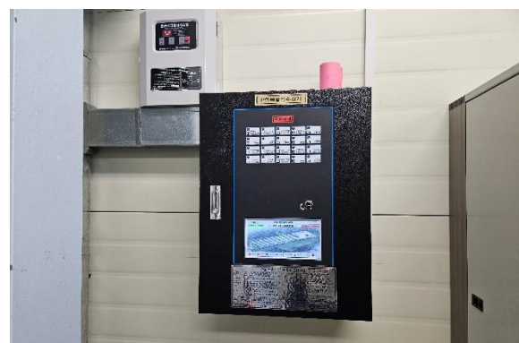
[Fire alarm control panel in the control room]
